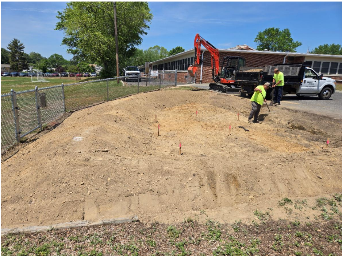
Rain garden installation at Pitman Memorial Elementary School, Gloucester County, NJ, May 2025 [Photo credit: Allison Nevulis]
